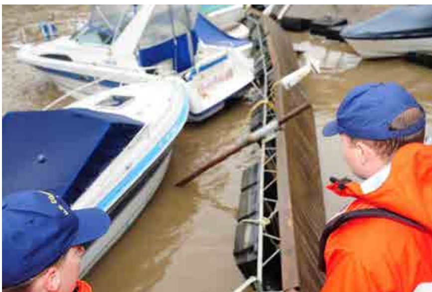
U.S. Coast Guard crews survey damage at a marina post-Hurricane Sandy (Photo: USCG)
